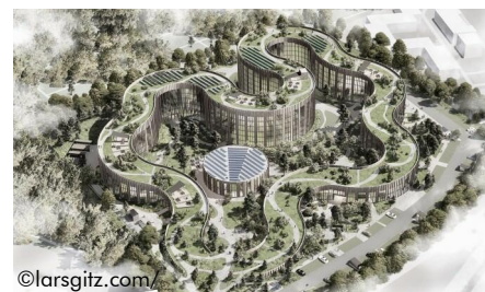
The large green roof buffers rainwater, reduces the ambient temperature, cleans the air and saves energy.
