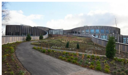
The path on the roof rises 22 meters from ground level to the highest point on top of the 6 th floor.
