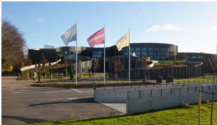
The modern student accommodation combines a unique design with a sustainable, innovative construction.
