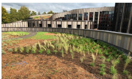
The substrate is applied in different heights to allow for a wide range of plants to thrive.
